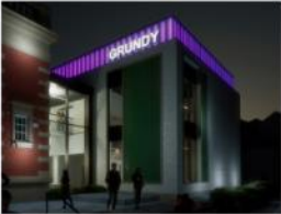
Opaque glass panels to form screening for rooftop plant areas. Illuminated to three sides only with variable colour output.
